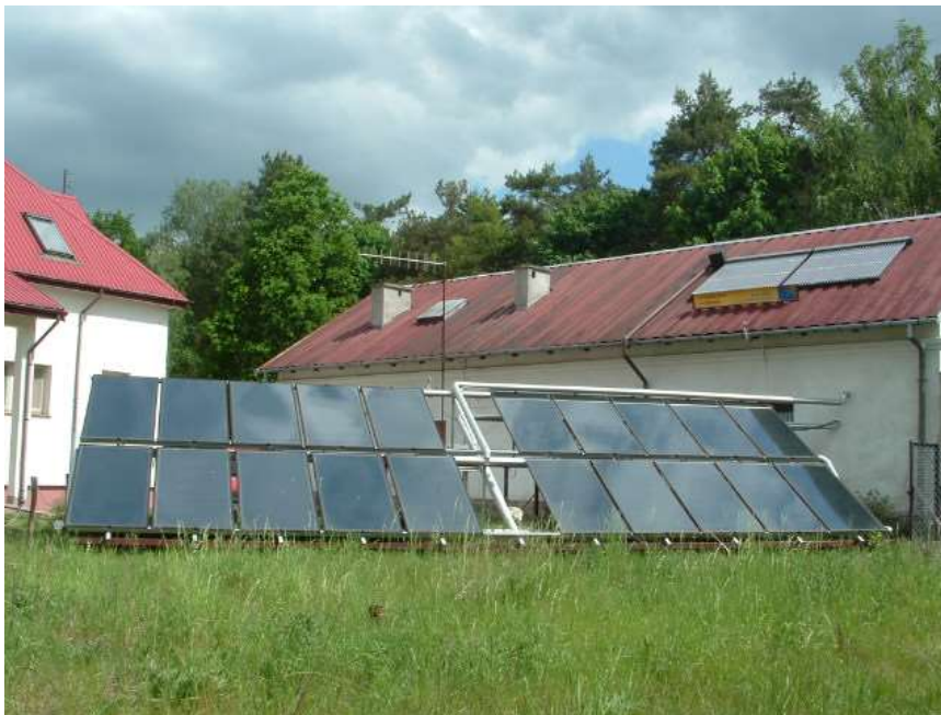
Fig. 2. The solar segments in the hybrid system
